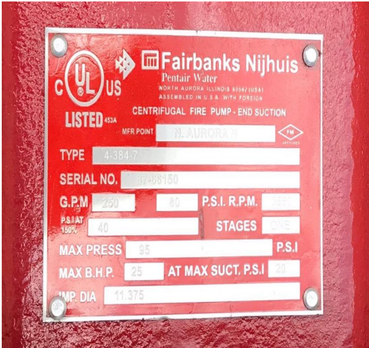
Figure 1 – Counterfeit Centrifugal Fire Pump Nameplate
